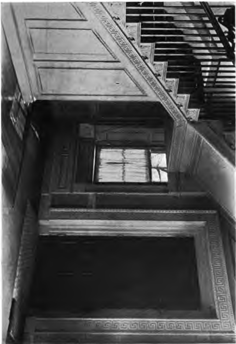
ENTRANCE HALL OF SCOTT HOUSE
